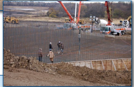
▶ This forest of rebar waiting for concrete is the emergency spillway below the dam as it looked in early November.
