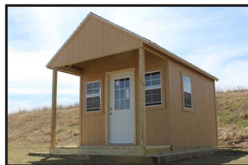
One of the cabins during construction
